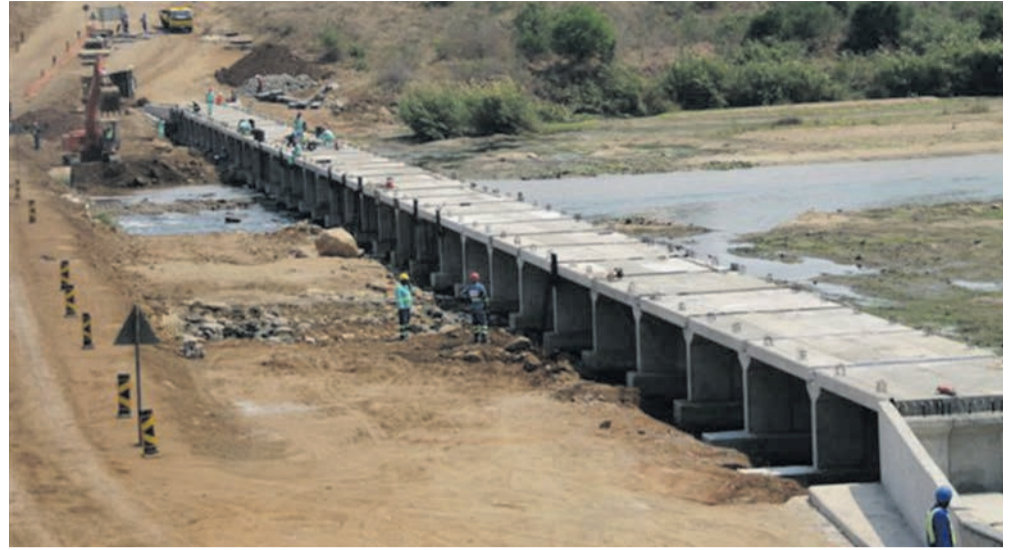
Crocodile Bridge under construction.
